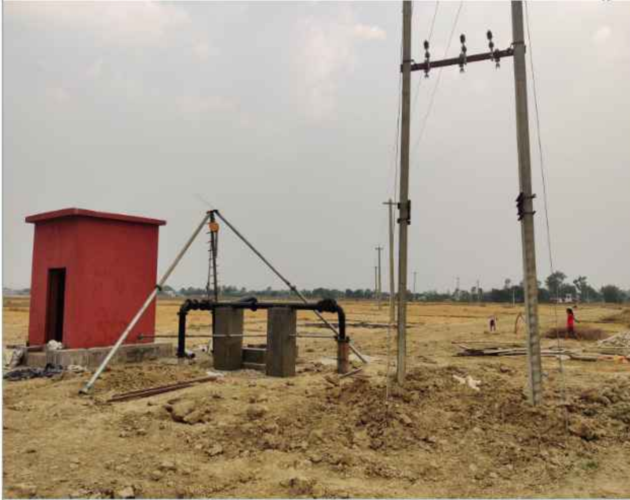
Pump House, MS Fitting, Electrical Items and Discharge of Neulapur Dtw Isp Thakurbaba Bardiya
